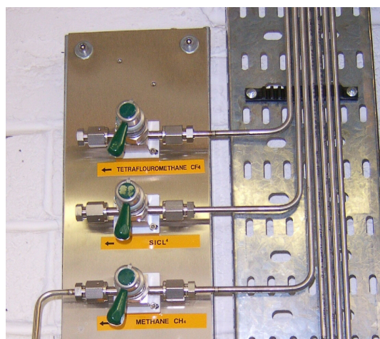
Figure 19 Gas supply point-of-use valves
